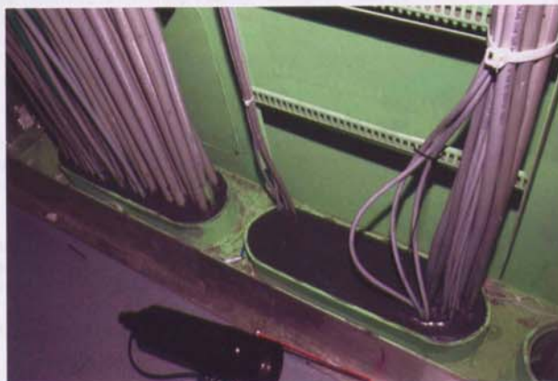
With the two-part RISE system, cables are passed through rubber insert sleeves and sealed with a silicone-based fire resistant and water repellent sealant
