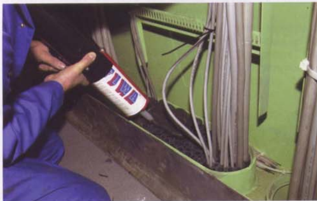
With the two-part RISE system, cables are passed through rubber insert sleeves and sealed with a silicone-based fire resistant and water repellent sealant
